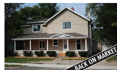
308 MAPLE • EAST JORDAN This 4BR home has been newly remodeled, has new flooring throughout and has been freshly painted. MLS 438295. Ask for Holly Nierman. $79,900
